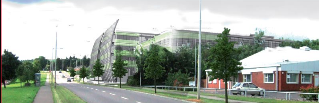
These before and after photos show how a proposed commercial development will sit in the landscape.
